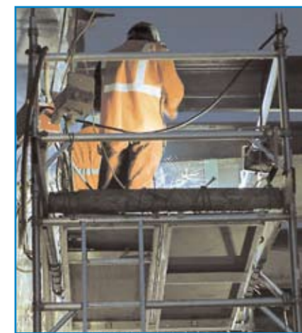
A scaffolding tower
