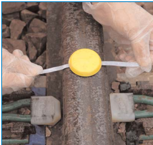
Detonator protection isn't placed at junctions
