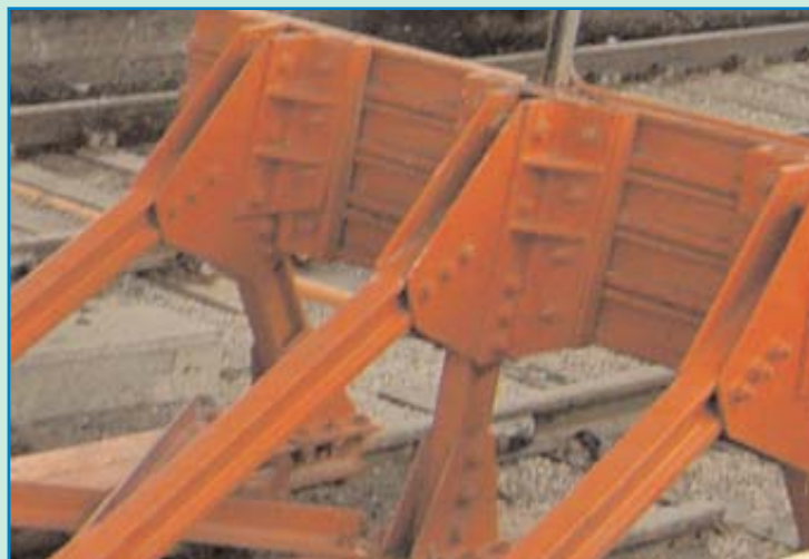
This buffer stop is adjacent to the mainline
