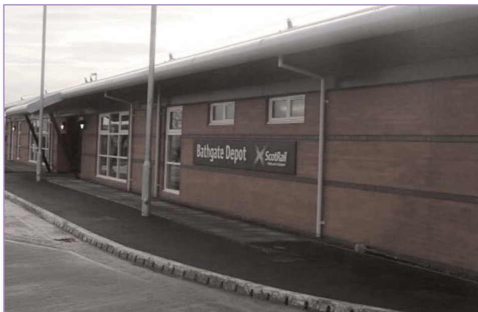
Pot holes on the route present slip, trip and fall hazards
