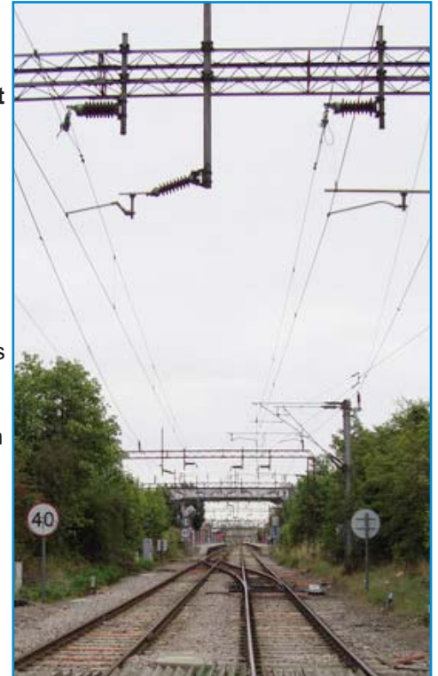
Network Rail inspected the entire Tilbury Line
