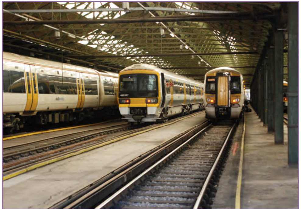
Grove Park depot sheds can contain unforeseen hazards
